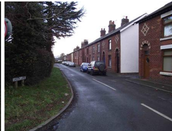
7. Terraced housing to Green Lane
