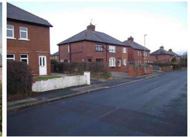
16. Existing 2 storey housing on Kepple Lane
